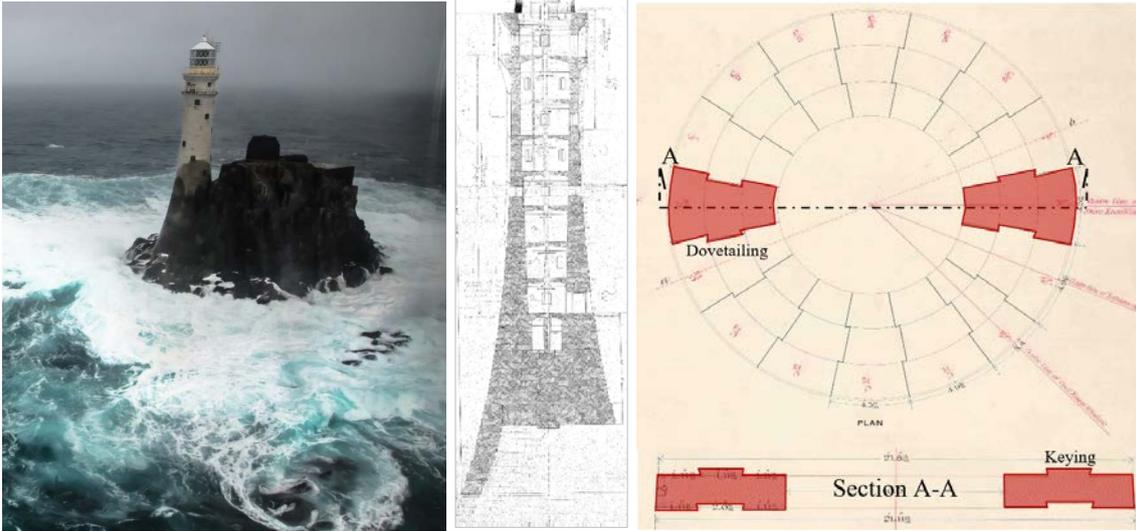
**Figure 1.** Fastnet lighthouse: (a) aerial photograph, (b) original section drawing and (c) details of dovetailing and keying for a course of stones.
