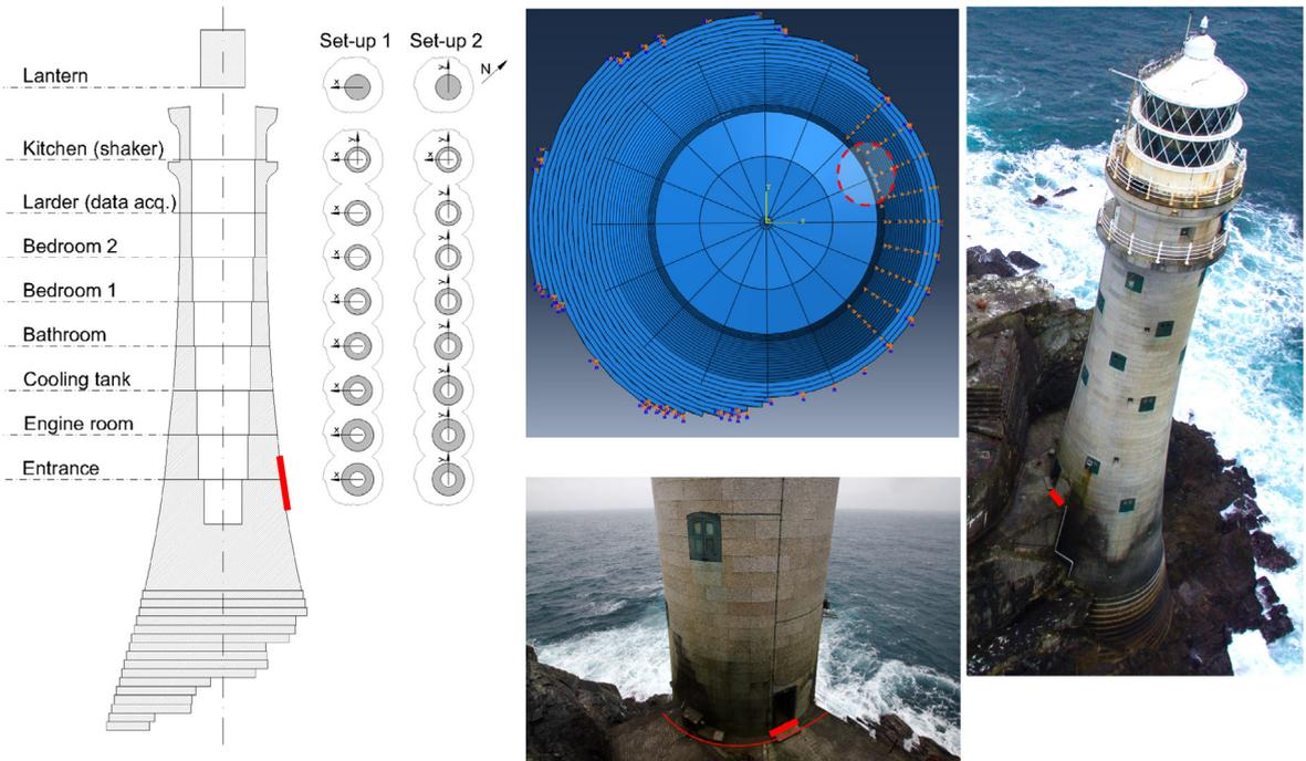
**Fig. 3.** Fastnet Lighthouse: (left) vertical section through structure and accelerometer arrangements in two sets, (mid upper) FEM showing door, (mid lower) view of rock restraint from stump of old tower, (right) drone view showing extended courses. Measurement x axis is through door, FEM x axis is rotated 22.5° clockwise from door. Photos: James Bassitt and Athanasios Pappas.
